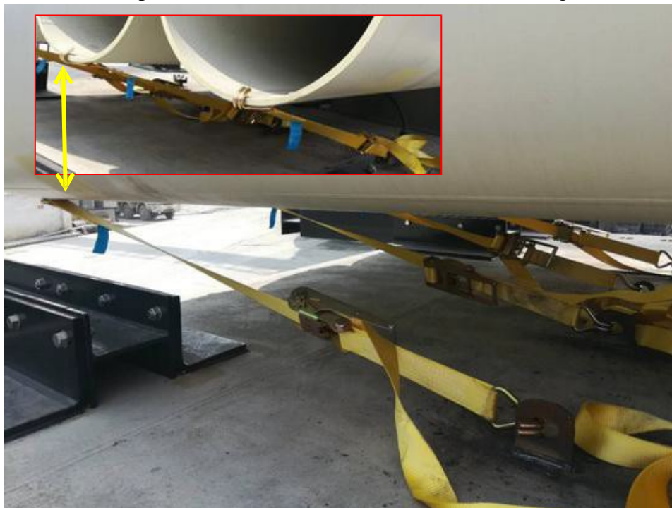
Pipe's another end was secured onto the deck ring
