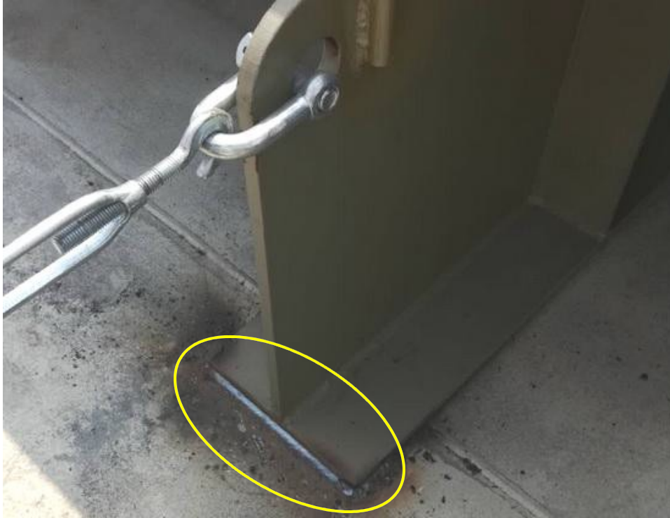
Cradles were secured and welded on deck
