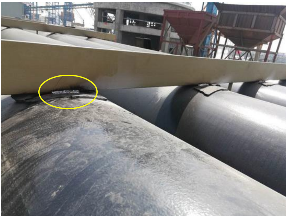
Pipes were welded on to the cradle's top angle steel
