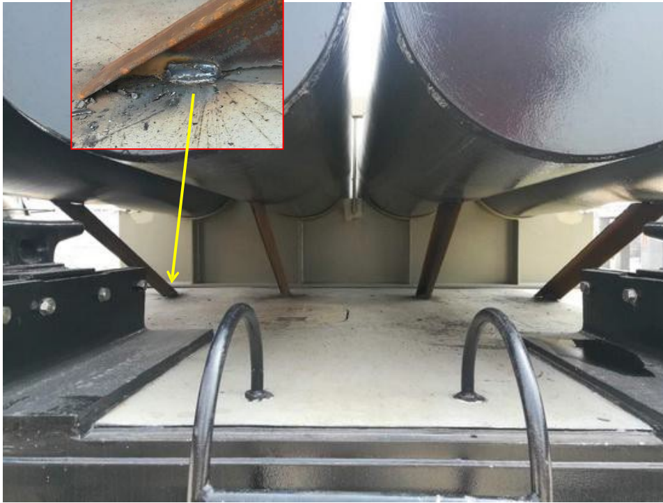
Pipe's one end was welded on to the deck with L type angle steel
